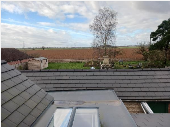
Left: View from upper floor west facing window
