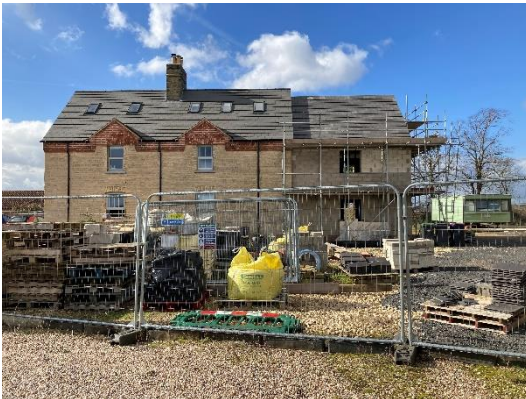
Left: Eastern elevation of properties
